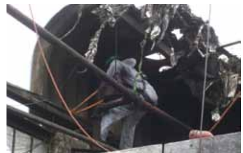
REMOVAL OF DEBRIS FROM FACTORY FIRE
