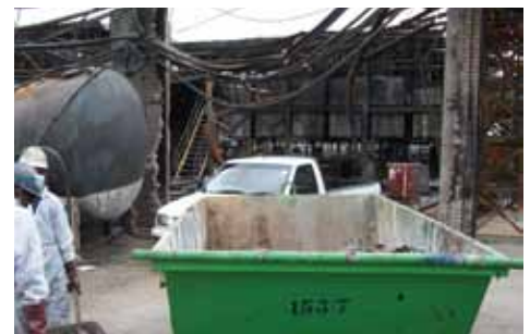
BURNED DEBRIS REMOVAL AND DISPOSAL
