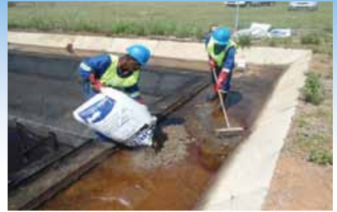
EFFLUENT OIL COLLECTION DAM CLEAN-UP
