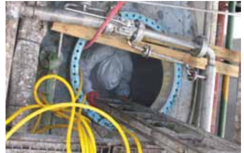
CHEMICAL TANK CLEAN-UP
