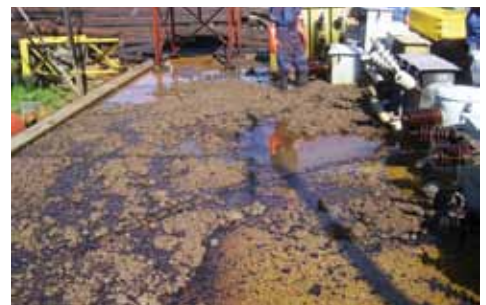
TRANSFORMER OIL STORAGE AREA CLEAN-UP
