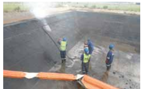
EFFLUENT CONTAINMENT DAM HIGH PRESSURE CLEANING
