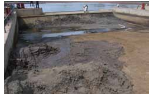
EFFLUENT SETTLING POND DESLUDGING
