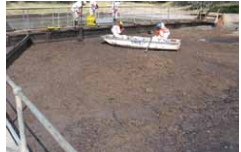
EFFLUENT DAM DESLUDGING AND CLEANING
