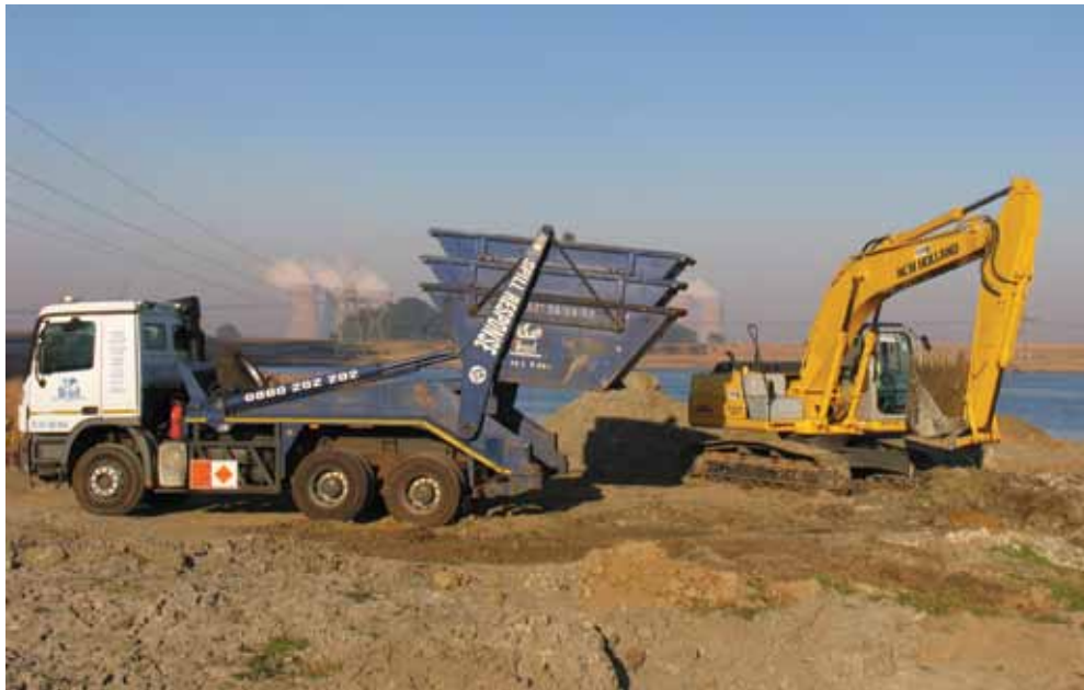
SKIP LOADER AND SKIP BINS
