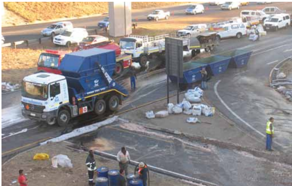
LARGE SCALE WASTE REMOVAL
