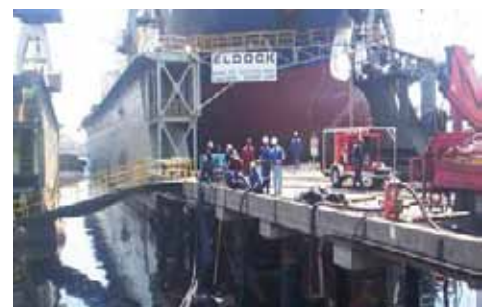
LEAKING VESSEL SPILL CLEAN-UP
